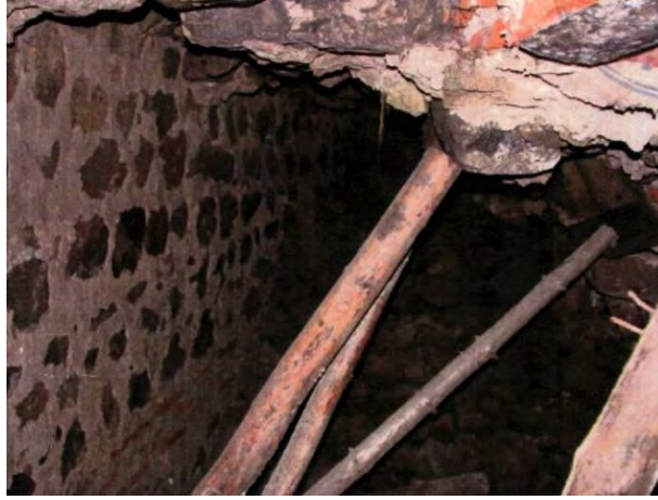
Figür 308: 1 Nolu Mekan
