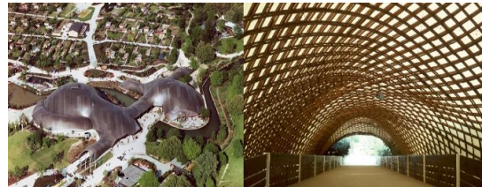
Multihalle Mannheim / Frei Otto / 1968. Source: Frei Otto, 1995.
