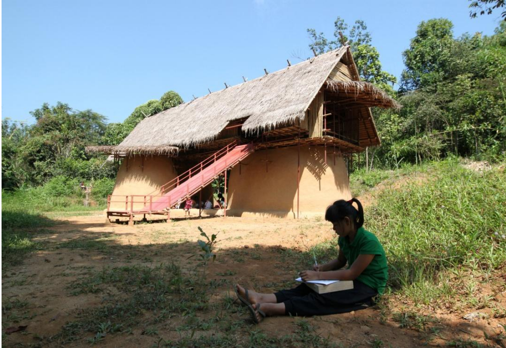
Görsel 5.10. Shangkhaburi Köy Okulu; https://www.archdaily.com/630188/floating-in-the-sky-school-for-orphans-kikuma-watanabe , erişim tarihi: Kasım 2018
