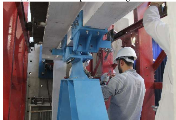
(d) Completed assembling of strengthening system
