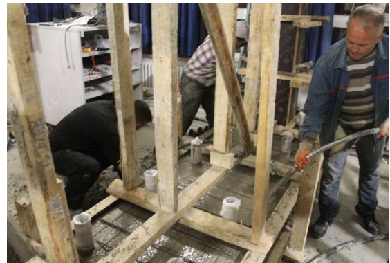
(b) Vibration process of concrete
