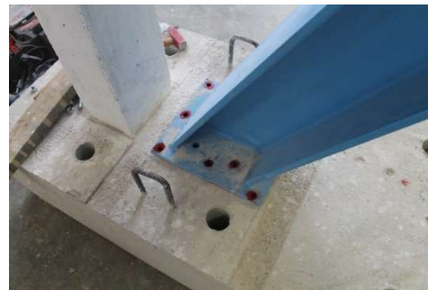
(b) Marking of holes with red color
