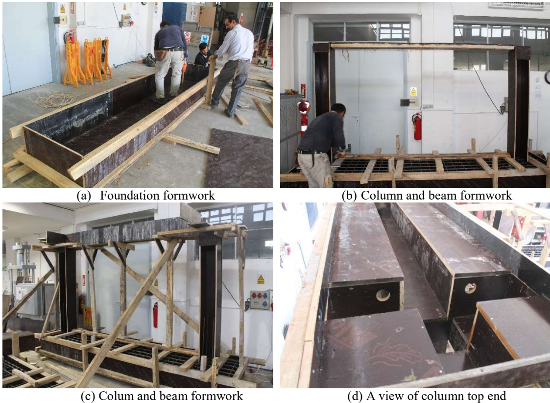
Figure 3.26. Formwork works
