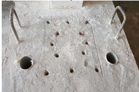
(c) Drilled holes on the foundation
