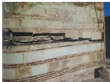
(b) Material decay on the wooden beam located in the South Wall
