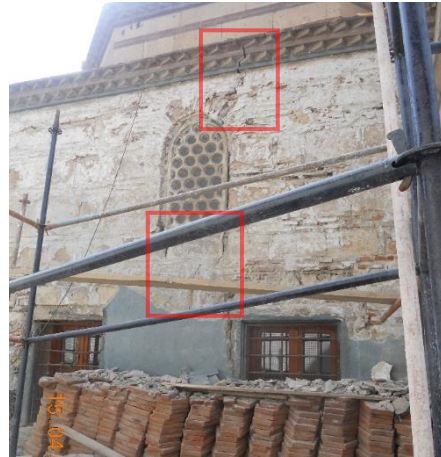
(b) East façade
