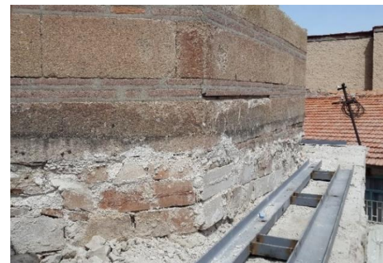
(d) Covering the girders with new masonry material
