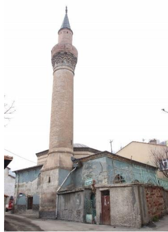
(a) North-East façade (Http-8)
