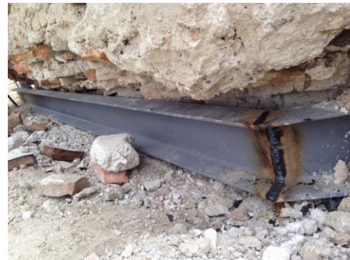
(b) Welded connection
