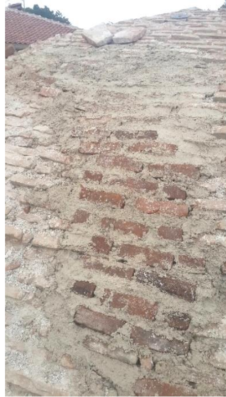
(e) Covering the steel elements
