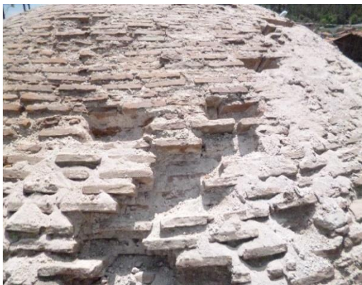
(a) Removing the old material
