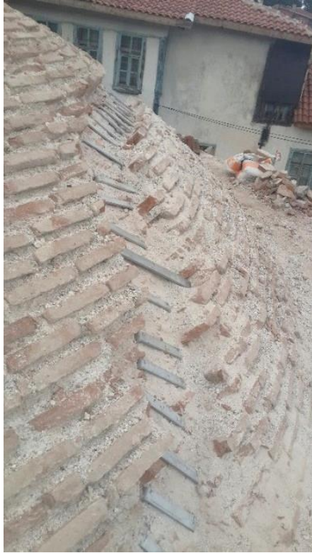
(c) Stainless steel elements fixed along the crack
