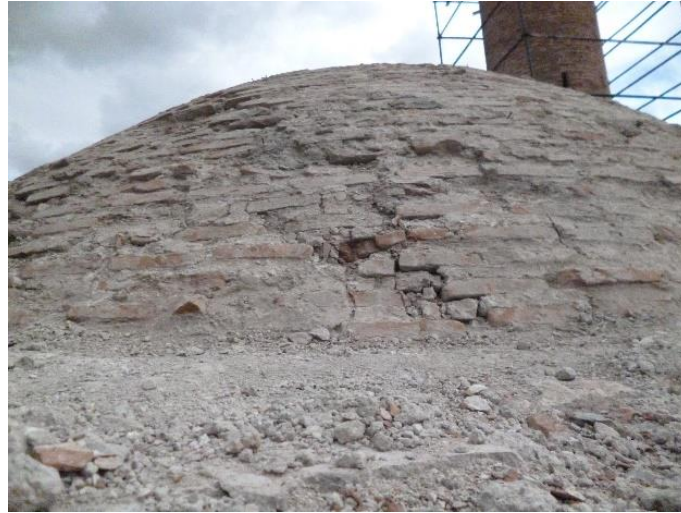
(a) Crack observed on the extrados
