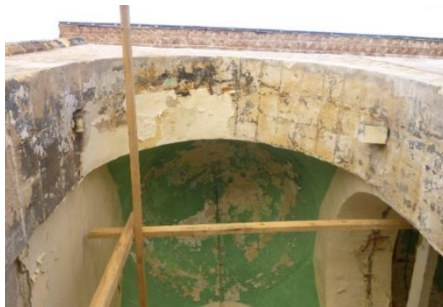
(a) Removed wooden tie beam
