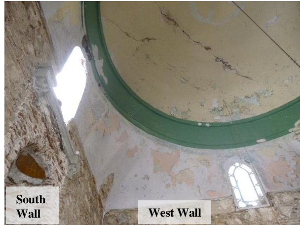
(a) Interior face of the south and west wall and intrados
