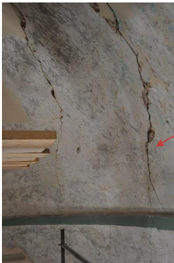
(b) Dome-drum-south wall
