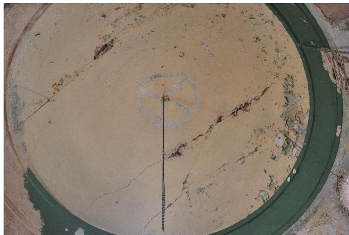
(a) Crack observed on the extrados
