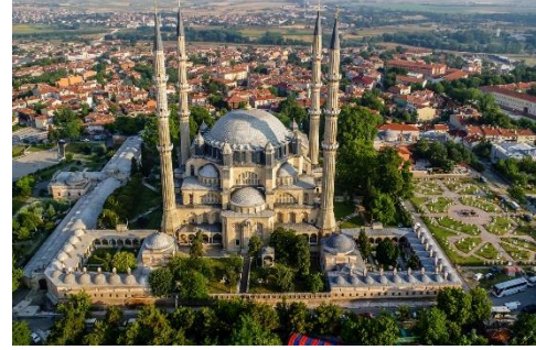
(b) Selimiye Mosque and its Social Complex
