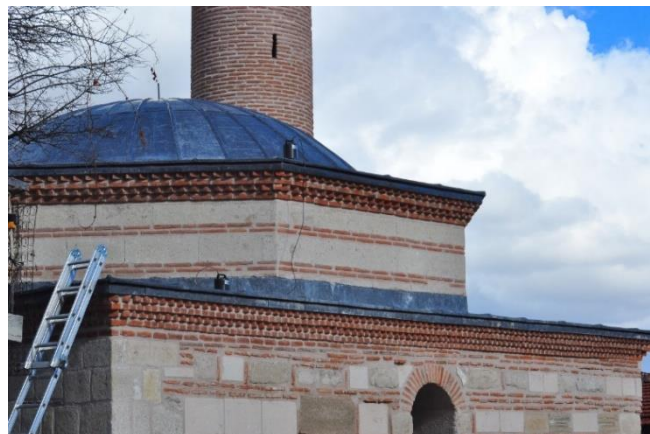
Figure 2.20. Lead covering after steel girder retrofitting
