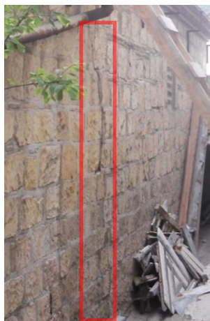
(a) Intersection of the Prayer Hall and Portico
