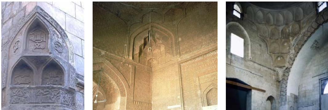
Figure 3.18. From Left to Right; Chamfered corner muqarnas of the Aqmar Mesjid (1125 CE) in Cairo (photo source: Wikipedia) , Masjid Jami (1105-1118 CE) or Friday Mesjid of Gulpayigan's squinch muqarnas ( https://archnet.org/sites/3872/media_contents/41008 ), Matbakh (kitchen) al Ajami (13 th c.) of Aleppo's pendentive muqarnas ( https://archnet.org/sites/10559/media_contents/111592 )
