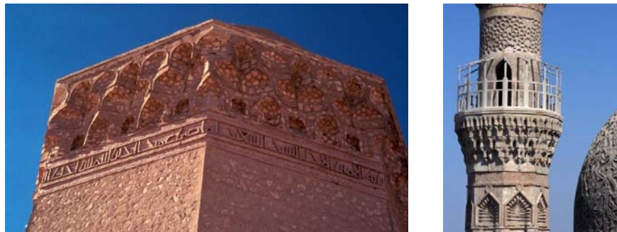
Figure 3.19. Left - Tomb tower of Gunbad-i 'Ali's cornice muqarnas (1056 CE) located Iran ( https://archnet.org/sites/1594/media_contents/975 ); Right - Amir Khayrbak Funerary Complex (1502CE) minaret balcony supports corbels, ( http://archnet.org/media_contents/46235 )
