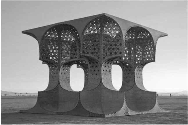
Figure 4.10. Muqarnas units scaled up to make self-standing structure (From the Burning Man Festival 2014, designed by Josh Haywood)
